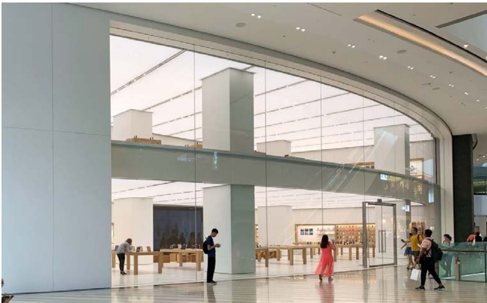
Fig. 5 Thermally toughened warm-bent (lamination-bent) glass fabricated by Sedak. Singapore Jewel Apple Store. Architects: Woods Bagot HK | Structural Engineers: Eckersley O'Callaghan | Contractor: Seele Austria.
