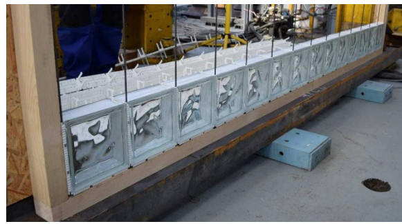
Fig. 3a) Assembling of the wall, a) assembled spacers ready to accommodate the blocks, b) the first row of the blocks is finished.
