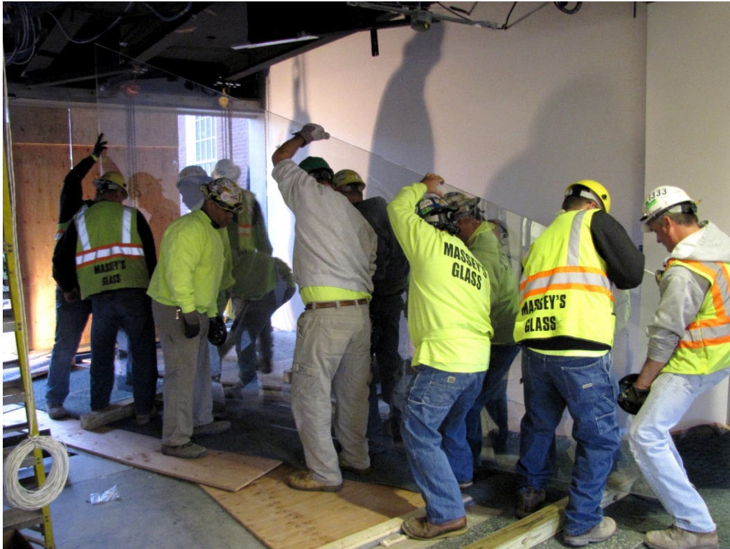
Fig. 8 P-131317, 2011 | Glass installation
