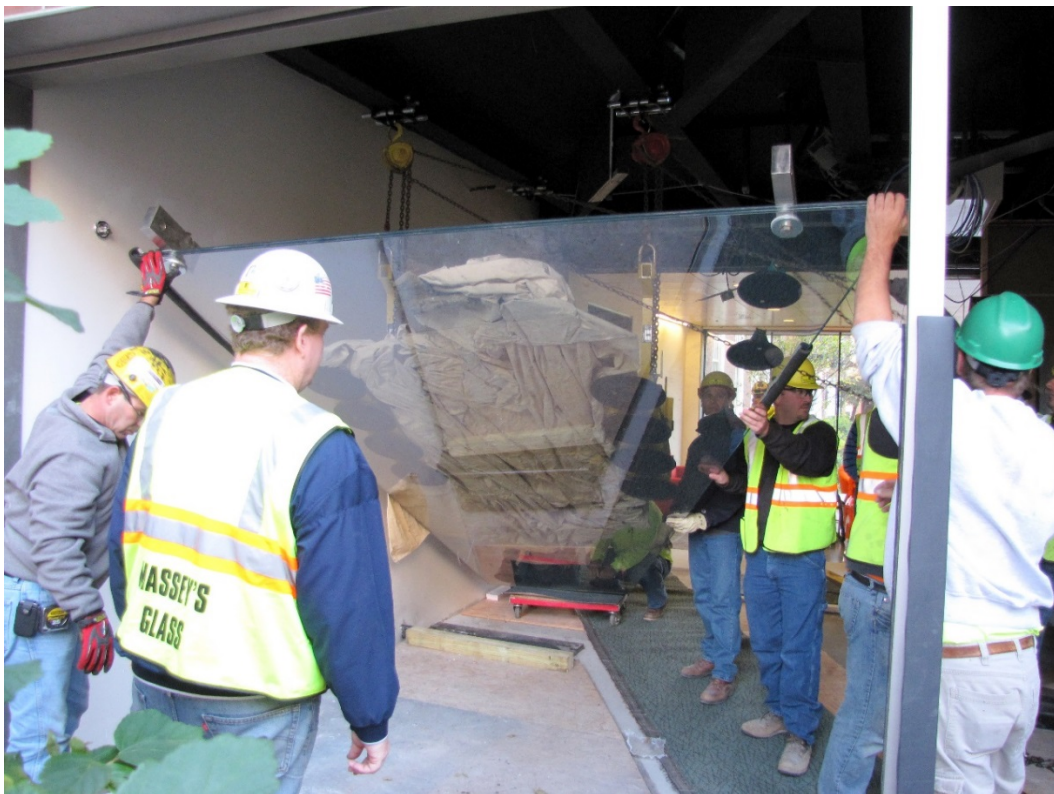
Fig. 9 P-131317, 2011 | Glass installation
