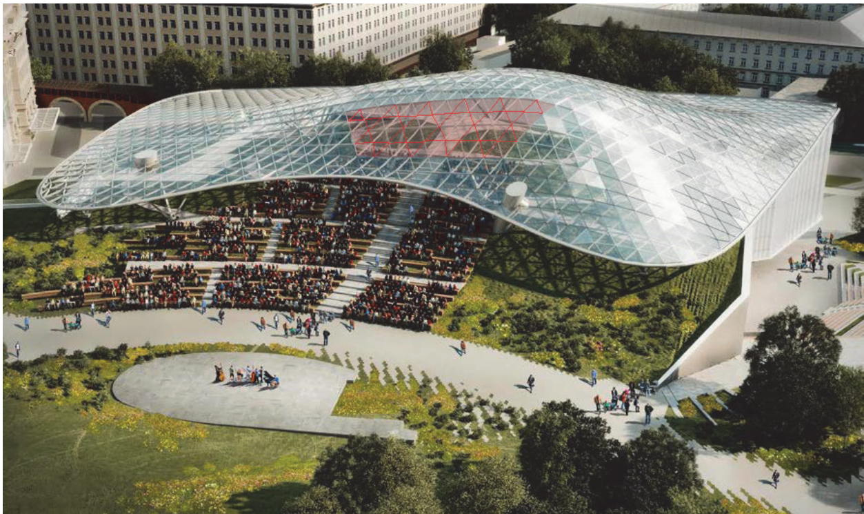
Fig. 1: General view of the canopy with area in question highlighted in red
