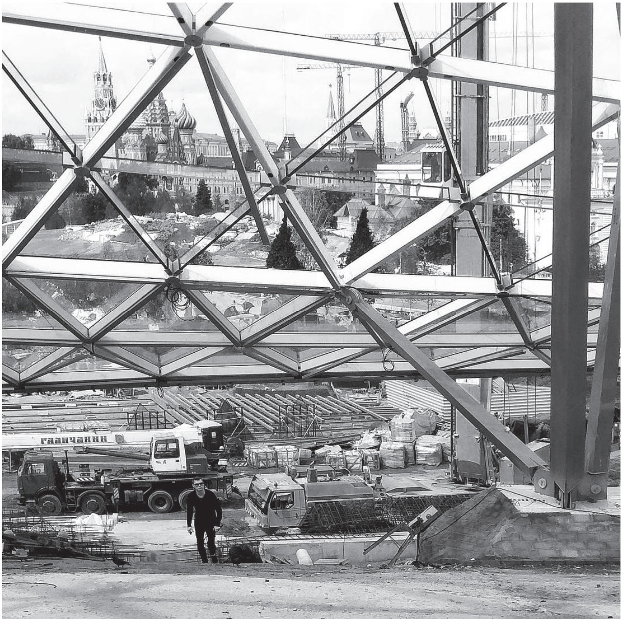
Zaryadye Park, Glass Grid Shell Roof
