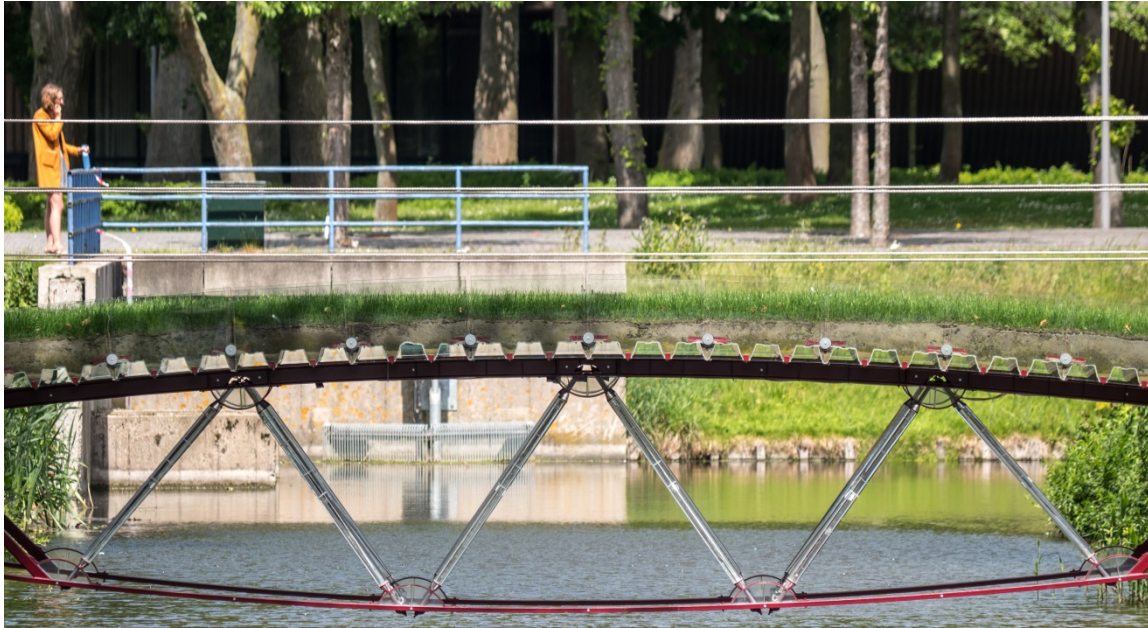
Fig. 2 photo of the glass truss bridge.
