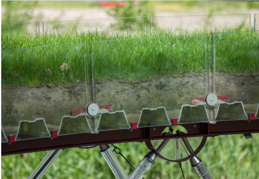
Fig. 4 Photo of detail of the glass truss bridge showing deck.
