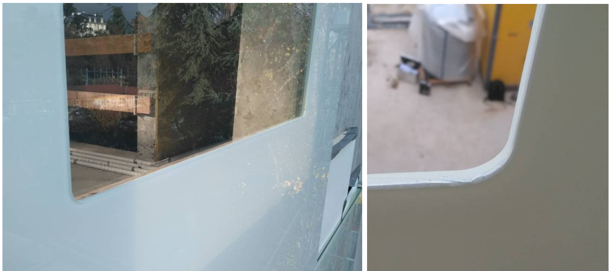
Fig. 11: Detail of pocket edge and PVB cut off quality for double skin zone
