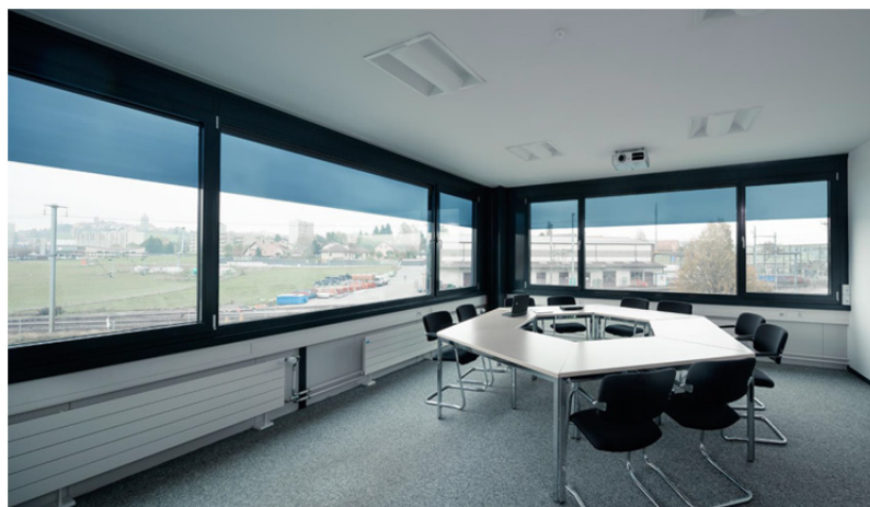
Fig. 7 Example of one of the new developments in EC glazing: in-pane zoning. This shows EC glass installed in a refurbished building in Switzerland with the top of each pane in a tinted state and the bottom in a clear state. ©Vetrotech Saint-Gobain.
