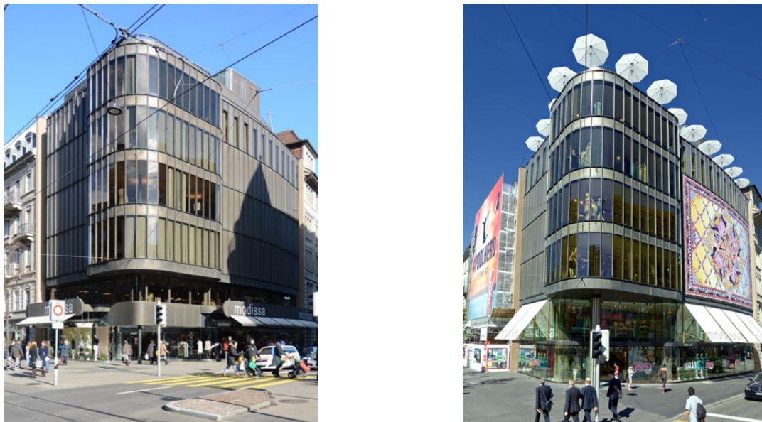
Fig. 8a) and b) The exterior façade of Modissa fashion store, before and after retrofit with EC glass. ©Vetrotech Saint-Gobain
