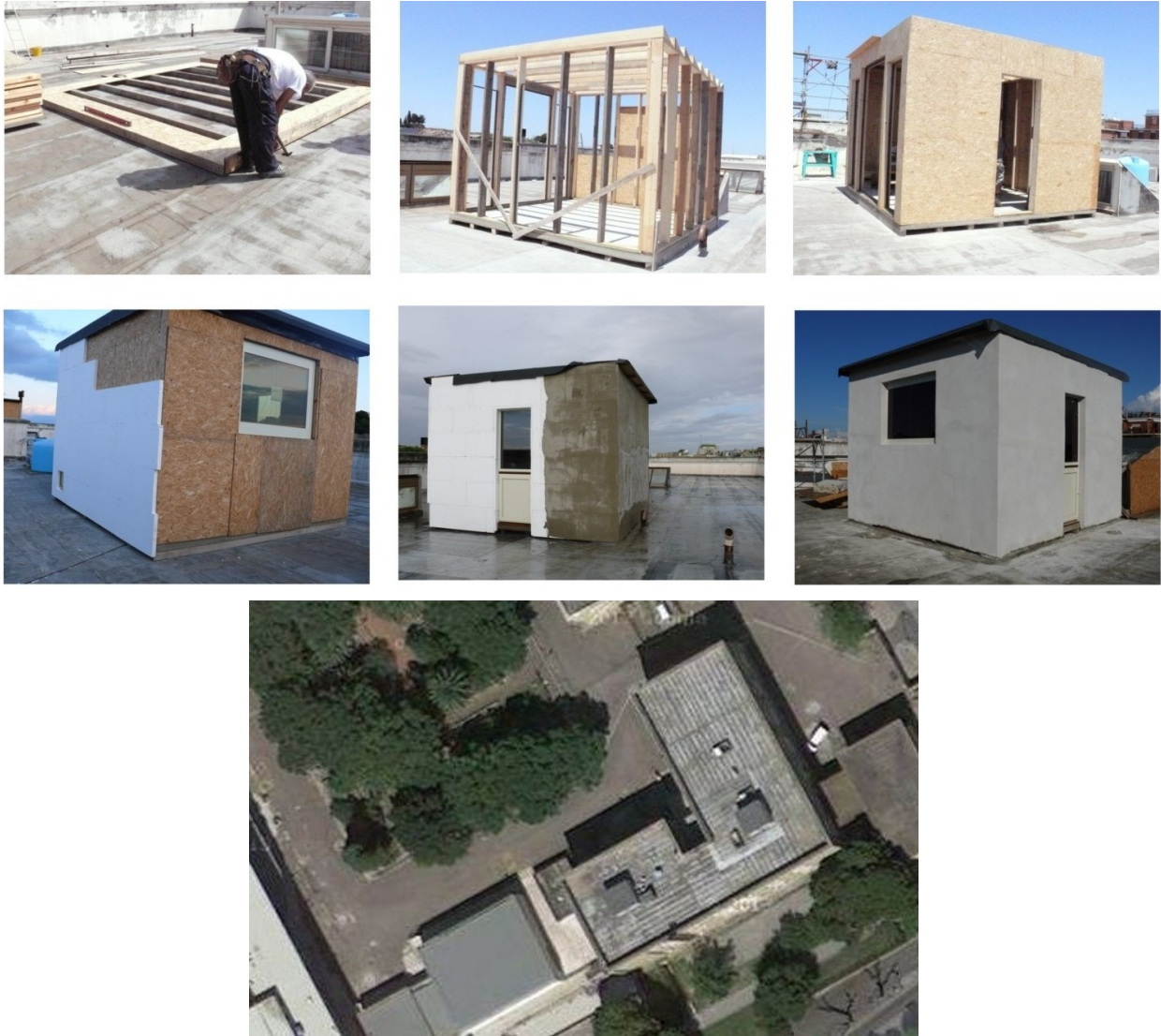
Fig. 1 Building phases and aerial view of the test rooms (July – November 2011).
