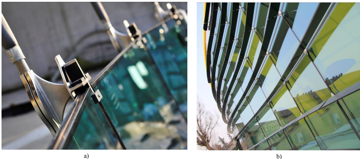
Fig. 9a) View of the glass fixing and cable clamp (Studio 129) 9b) View of the façade with sun shading elements (Studio 129)
