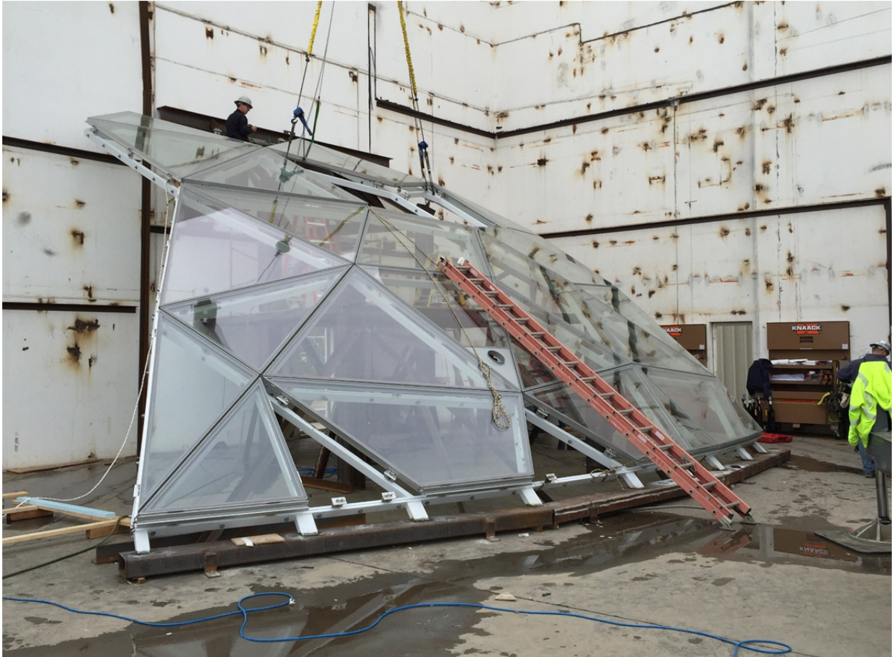
Fig. 10 Construction of Multi-faceted Façade Performance Mockup.
