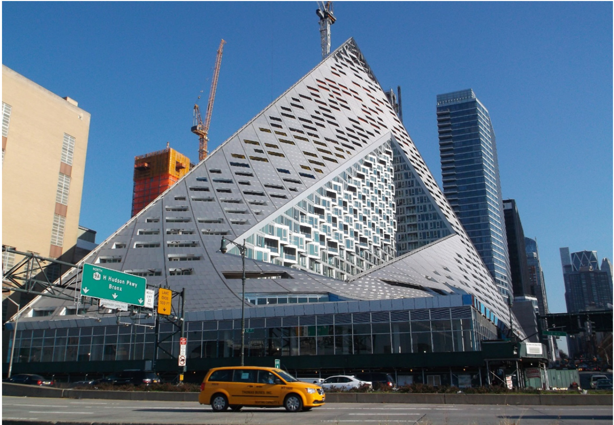
Fig. 2 Sloped Façade Construction as of November 2015.
