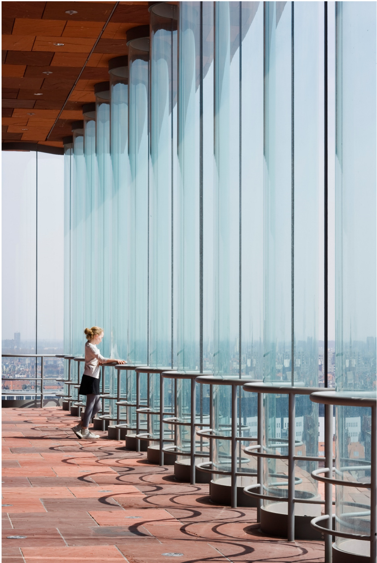
Fig. 5 MAS Museum, inside view of corrugated glass facade. Photography Sarah Blee © Neutelings Riedijk Architecten.
