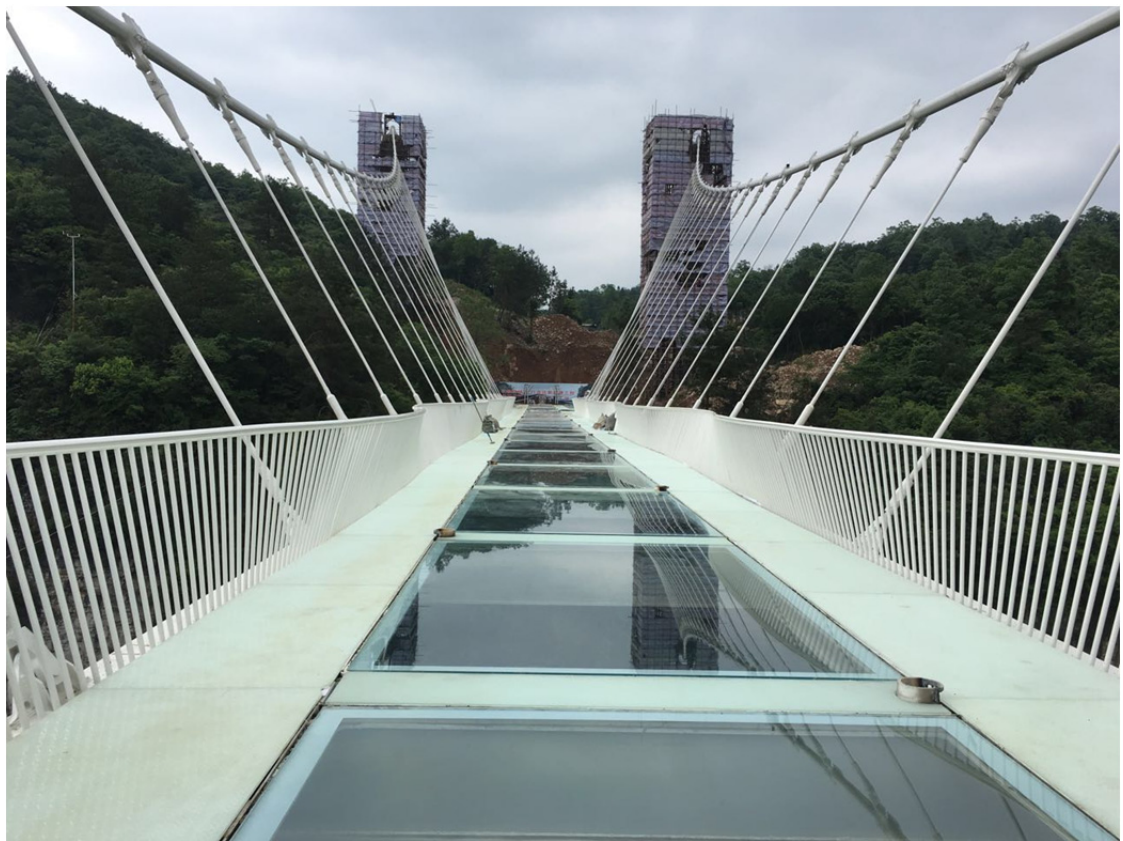
Fig. 9 Zhangjiajie bridge, view from deck..
