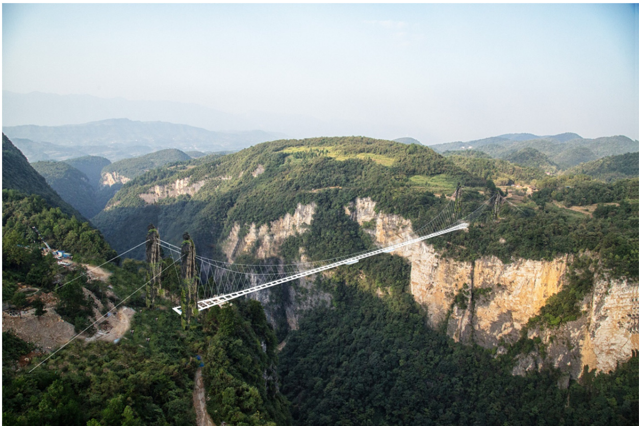
Fig. 1 Zhangjiajie Bridge, aerial view 1.
