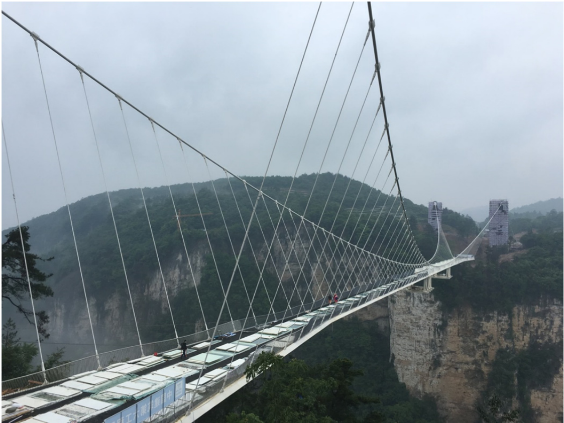
Fig. 9 Zhangjiajie bridge under construction, side view.
