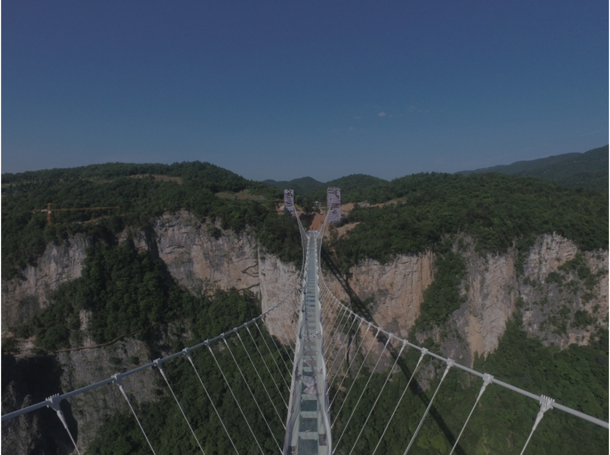
Fig. 5 Zhangjiajie bridge, view over the bridge.
