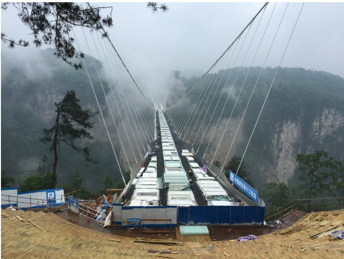
Fig. 8 Zhangjiajie bridge under construction, front view.
