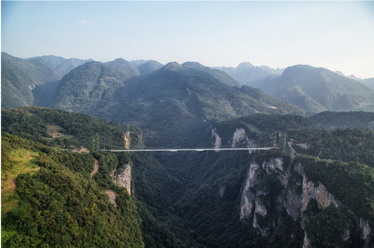
Fig. 4 Zhangjiajie bridge, aerial view 2.
