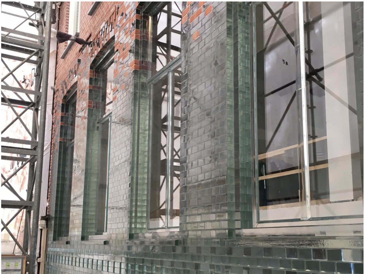
Fig. 10 The façade after the bonding and sealing of the ceramic tiles
