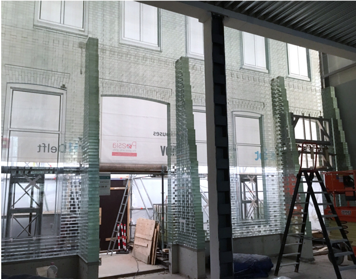
Fig. 16 The glass masonry façade.
