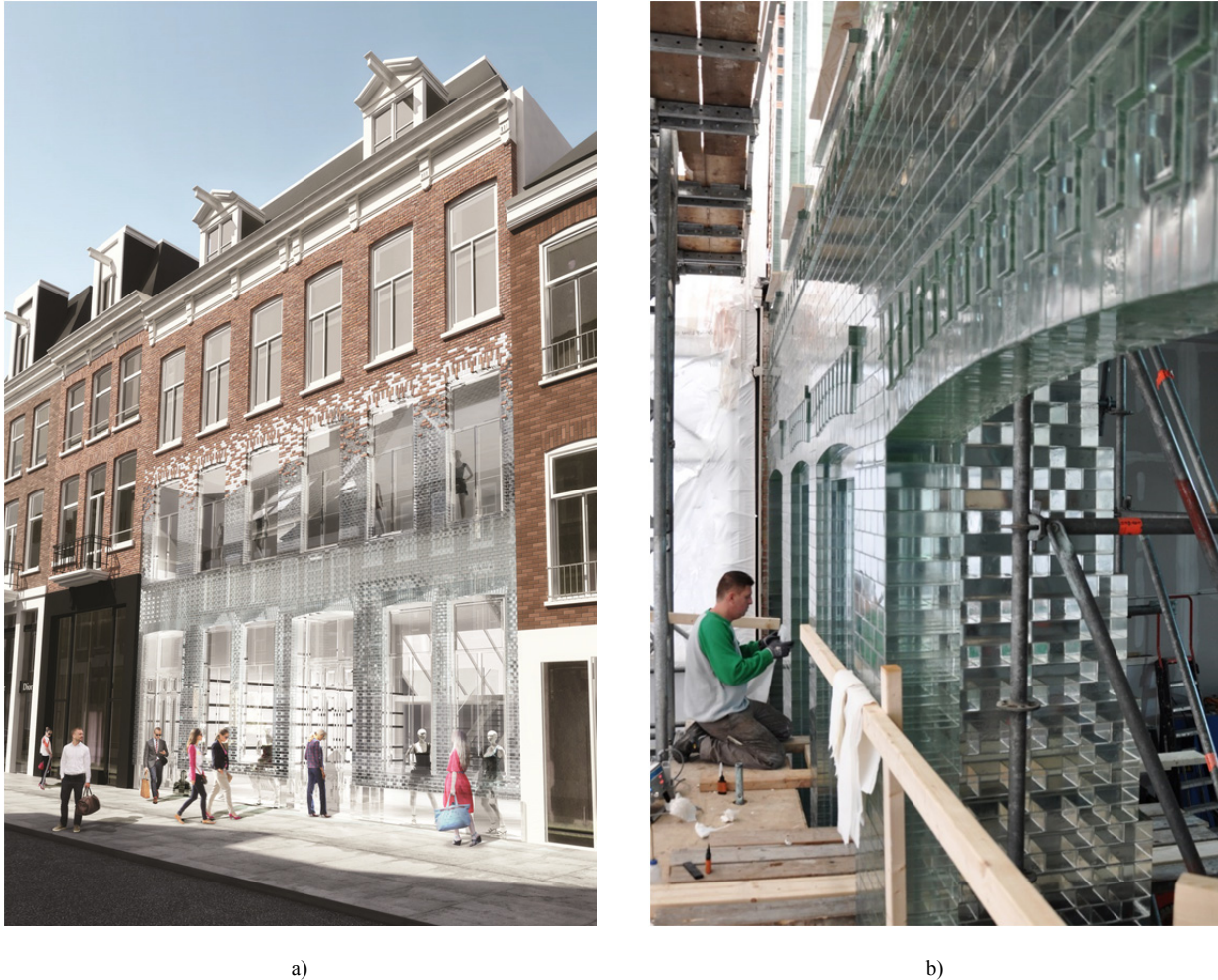
Fig. 2. a) 3-D impression of the glass block façade; b) Photograph of the façade during construction.
