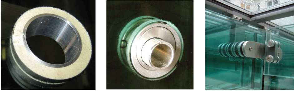
Figure 1a, b and c: Mortar-Interlayer to create ductility behaviour and example of a joint (CCI Munich)
