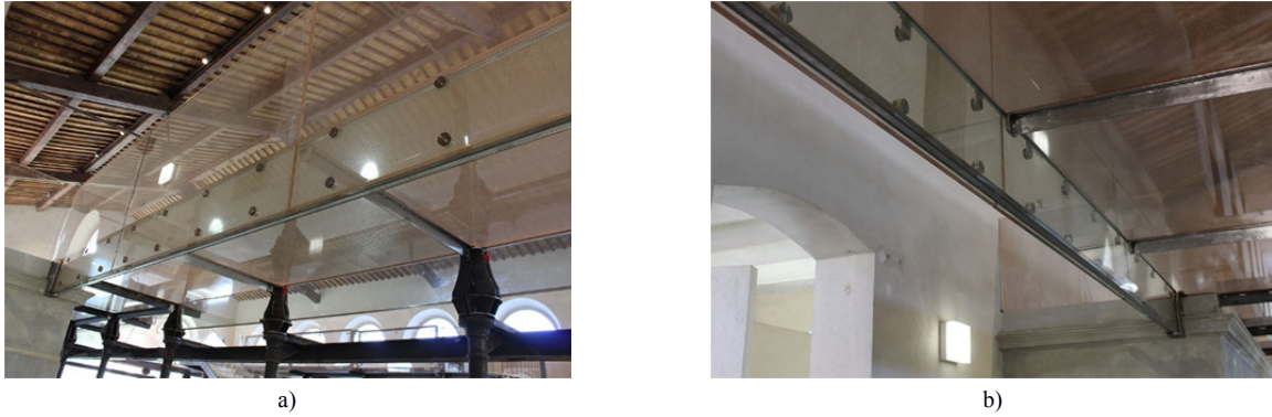
Fig. 2a) and b) The steel-reinforced laminated glass beam viewed from different positions.
