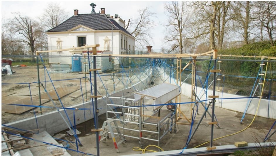
Fig. 14 The central hall of the pavilion under construction.
