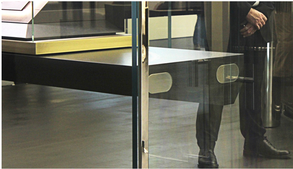
Fig. 12 High transparent TSSA glued connection of a show case to a full glass structure in an exhibition stand.
