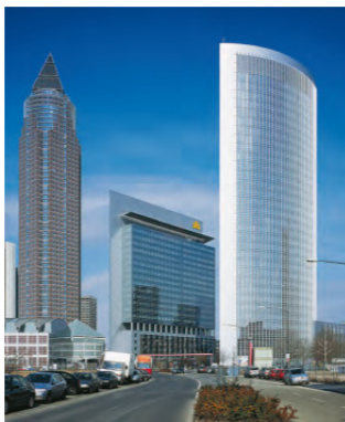
Fig. 1 Two sided structural sealant glazing system, Pollux and Castor towers in Frankfurt/Main, Germany (Dow Corning 2010)
