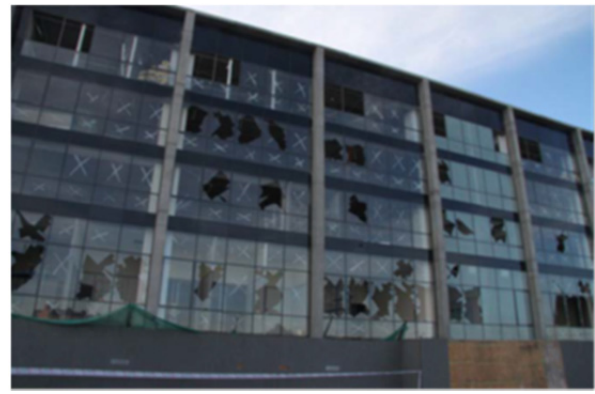
Fig. 3 a) Broken glass and bent mullions in flexible building which experienced large interstorey drift in Northridge (California) earthquake in 1994 b) Glazing damage in building in central Chile following 2010 earthquake (FEMA E-74, 2012).
